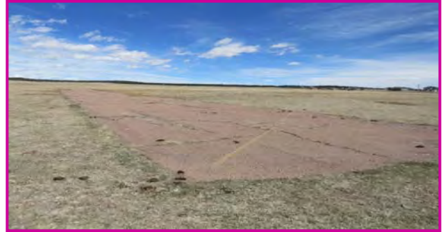
“The Closed Runway marking can barely be seen.”
